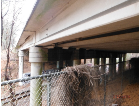
Photo 1. East Side View of bridge
