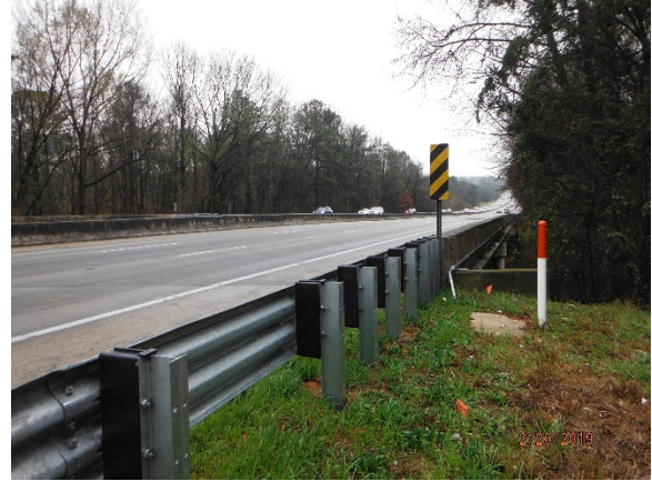
Photo 2. Top of Bridge Deck View
