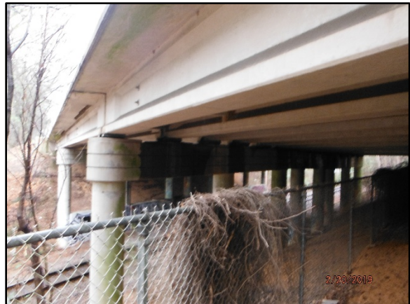
Photo 1 – I-20 Bridge over CSX Railway in Lexington, SC.
