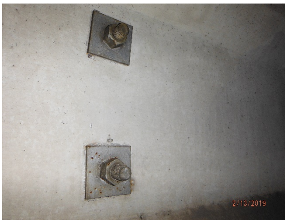
Photo 5. LBP Tie Rod Plates
